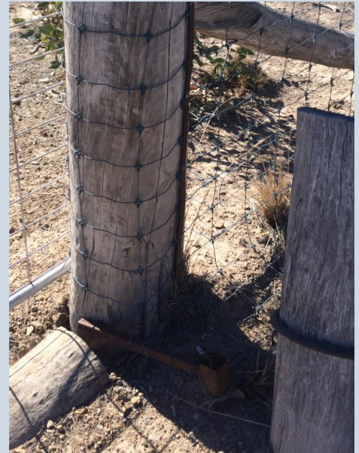
Staining the apron
